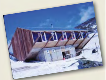
Yaraandoo during first stage construction 1962 (Photo: Courtesy of Yaraandoo Sk Lodge).
