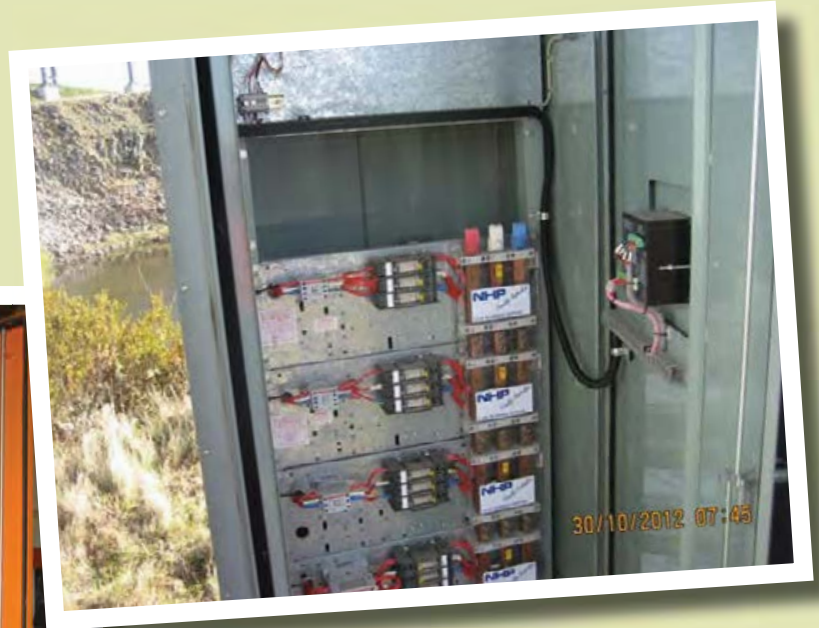
Mount Selwyn Snowfields Power Correction Unit (Photo: Courtesy of Mout Selwyn Snowfields).
