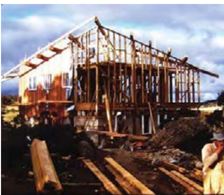
Ku-ring-gai Alpine Lodge under construction - Summer 1961-2
