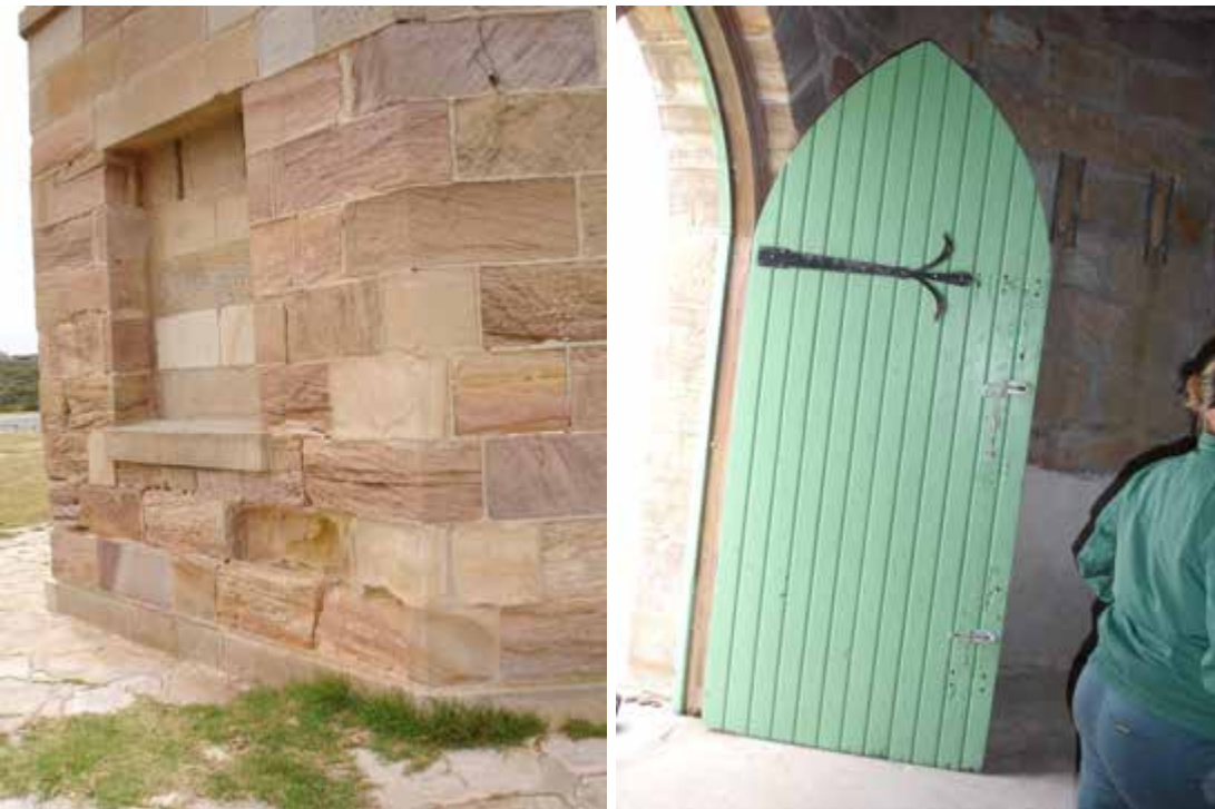
Fig. 5 (left) The degraded surfaces of the west facet of the octagon showing the abraded sandstone and the areas of missing and weathered mortar. Note also the concrete sills and infilled window openings. (Photograph by Sheppard, October 2006)
