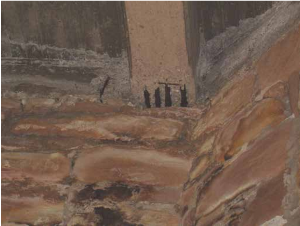
Fig. 4 The west end of the hanging concrete beam under concrete slab roof, showing the exposed and rusting reinforcing rods. (Photograph by Sheppard, October 2006)
