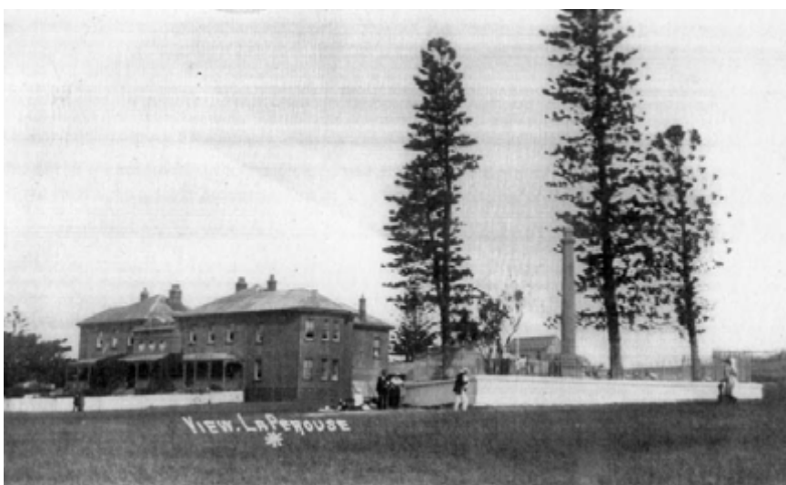
Fig. 6.13 View of the La Perouse Monument with Cable Station building in the distance. Tentatively dated 1906-1917 (Tuck: 174).
