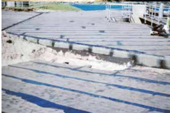
Figure 29. View showing the level change of the waterproofing membrane between Gun No.2 emplacement (lower) and the casemate water catchment area (higher).
