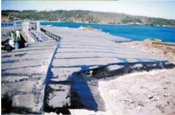
Figure 31. View of the casemate opening. The step in the concrete catchment area can be seen (dark seam at the left).
