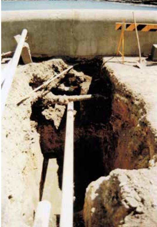
Figure 34. Photograph showing new piping laid in the pit. [Photograph and information courtesy of Greg Bond]
