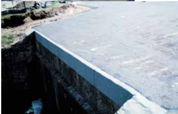
Figure 19. View looking south west indicating capping of waterproof membrane at the embrasure wall at the arc-of-fire. As can be seen no drainage method has been included to reduce water runoff from the waterproofed area onto the face of the iron embrasure wall.
