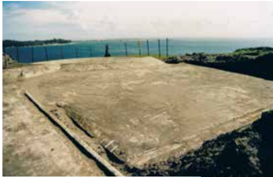
Figure 26. View of the roof area at Gun No.2 emplacement prior to waterproofing membrane being laid.
