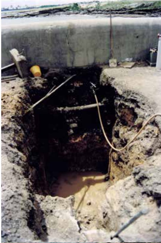
Figure 33. View of pit dug at western fortification wall at the entry forecourt in anticipation of installing a detention tank for water runoff. [Photograph and information courtesy of Greg Bond]
