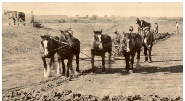
Figure 2.32 Making a ground tank, the horses are pulling a plough. Source: Yanga Archives
