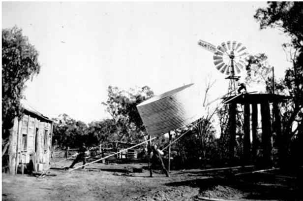
Figure 2.37 Raising a water tank onto an elevated tankstand, Waugorah 1925. Source: Museum of Victoria
