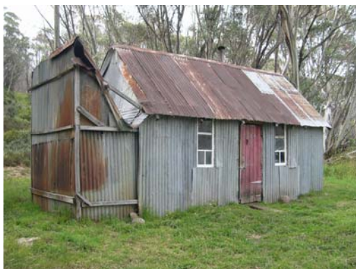
Photo 3.5.4.5a&b below Horse Camp Hut and toilet
