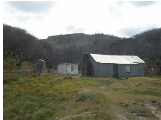
Photo 3.5.4.4a,b,c Whites River Hut toilet building, rear of toilet and Hut.
