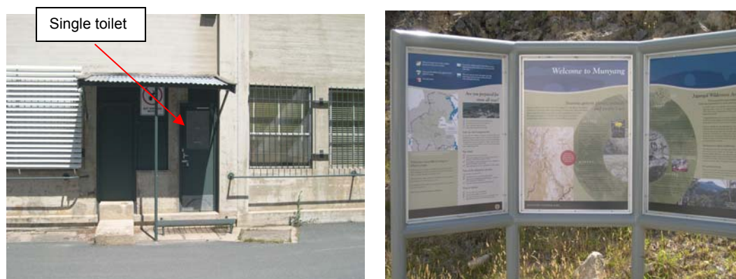
Photo 3.5.3.2a&b Guthega Power Station toilet and signage with Minimal Impact Code
