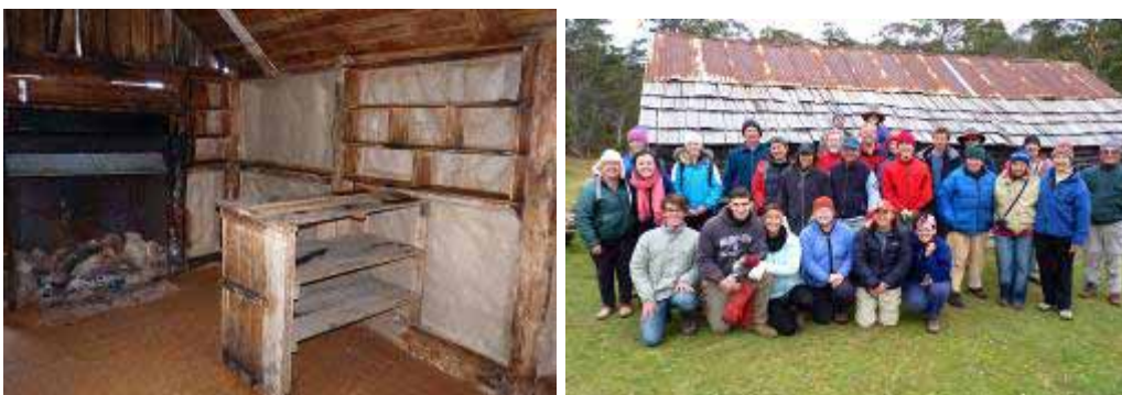
Refurbished interior and new rammed earth floor for the manager's hut at the Tin Mines(L). The impressive attendance at the 2012 Easter work party from the Illawarra Alpine Club at the Tin Mines (R). Photos: Rhonda Boxwell (Illawarra Alpine Club)
