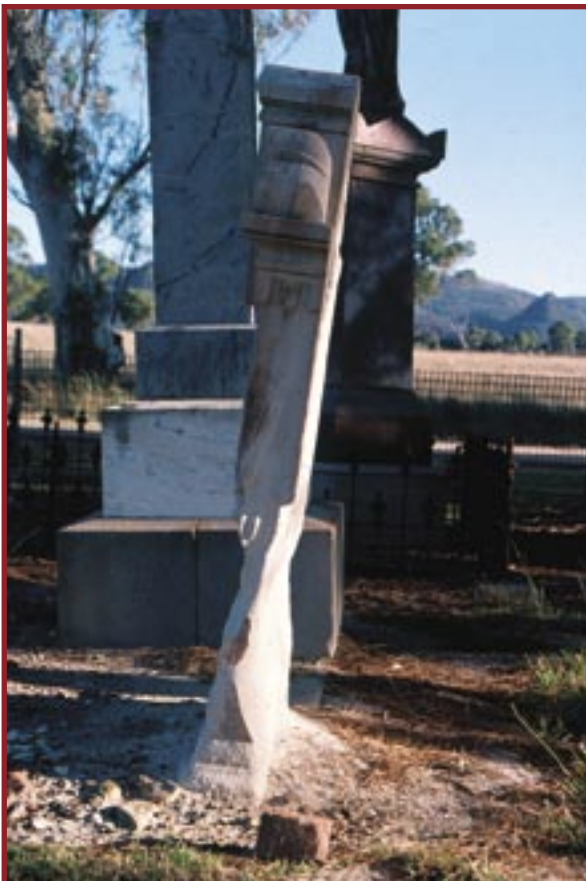
A headstone affected by salt and water. Photo: DIPNR
