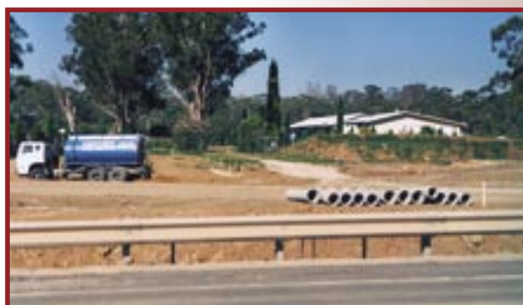
Road Construction can cause salinity problems. Photo: DIPNR
