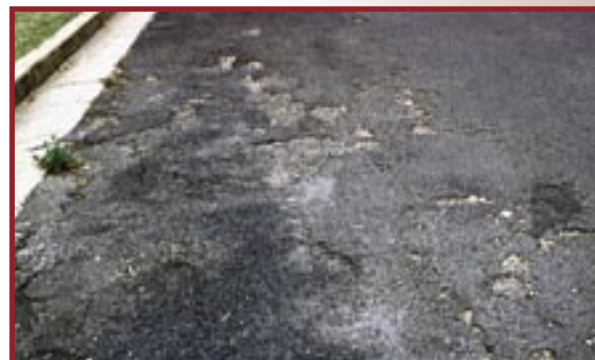
A road showing signs of salt and water impacts. Photo: DIPNR
