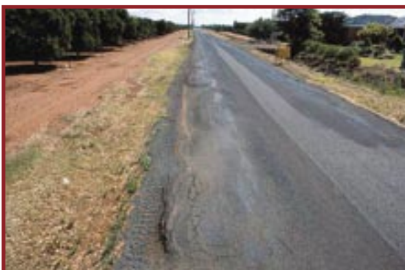
A road showing signs of salt and water impacts. Photo: NSW Department of Primary Industries
