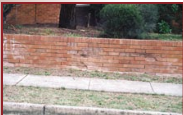
Bricks showing signs of salt and water damage. Photo: DIPNR
