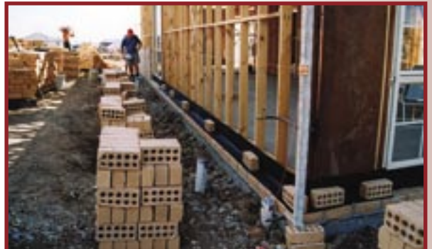
The installation of a damp proof-course. Photo: DIPNR
