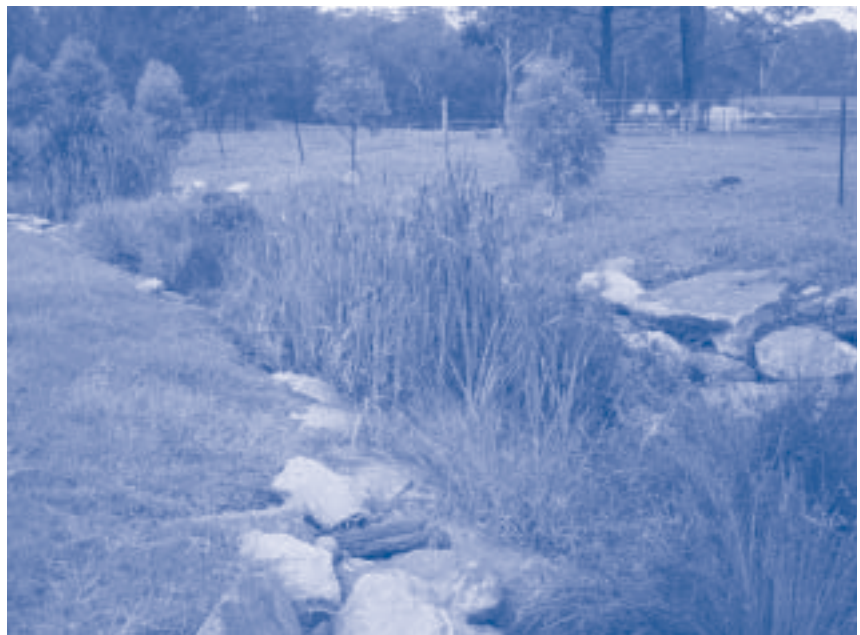
Wetland constructed to manage stormwater runoff.
