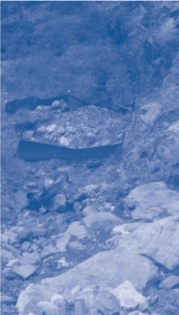
Before rehabilitation works
