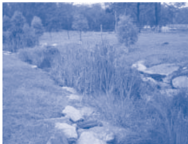
Wetland constructed to manage stormwater runoff.
