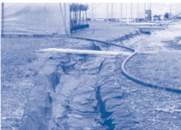
Drainage line improvement measures to reduce erosion along drainage lines.
