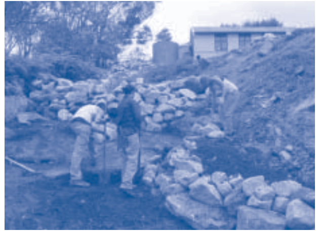
During rehabilitation works
