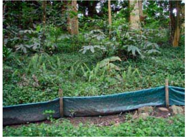
Figure 24: A sediment fence Photo: Nicholas Coleman
