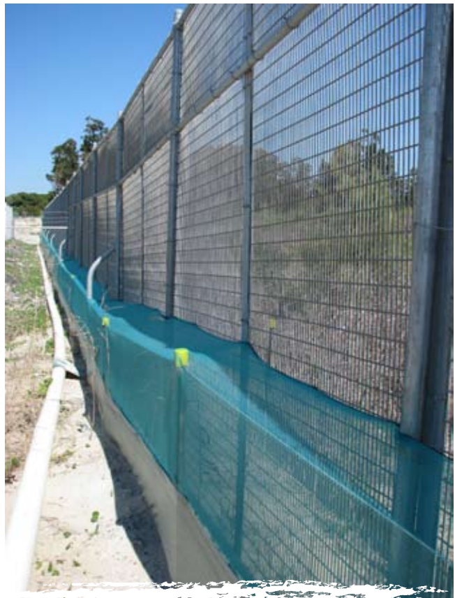
Figure 20: An example of a frog-proof fence against an existing cyclone fence at the Kurnell Desalination Plant
