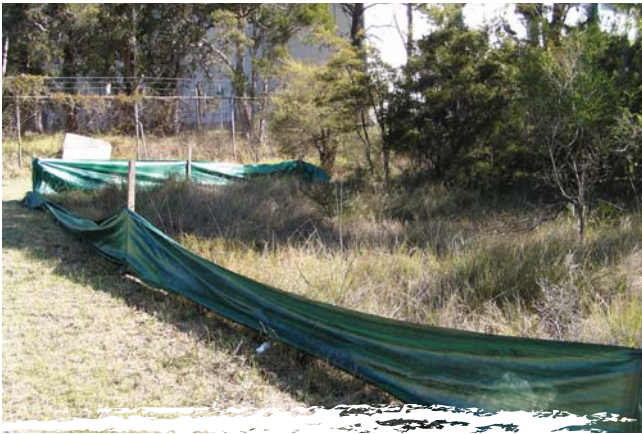
Figure 11: Sediment fence weed barrier in place
