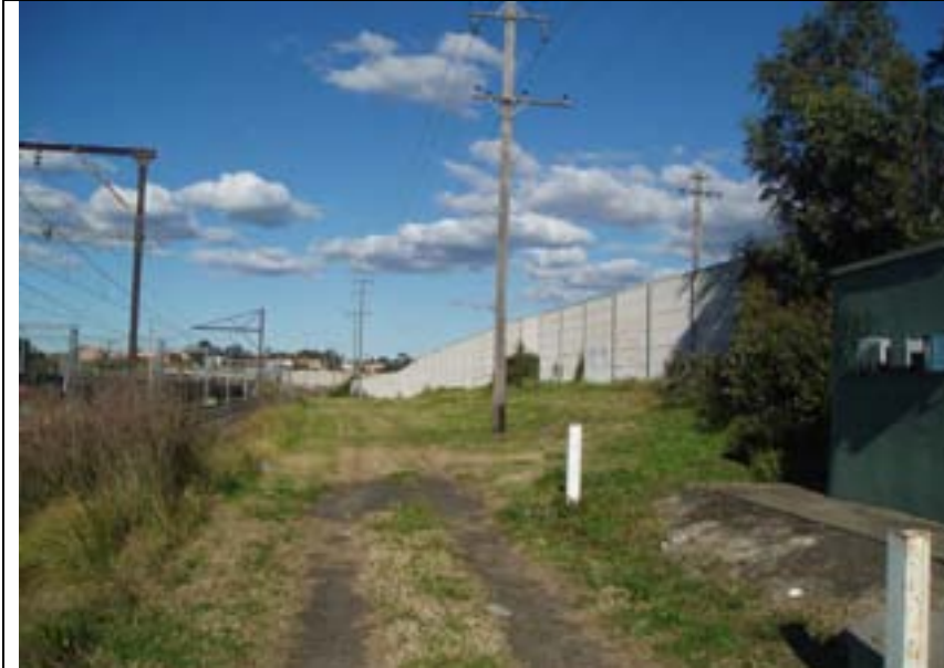
Sound barrier separating the Pacific National ponds and Hannas GGBF ponds (R. Wellington)
