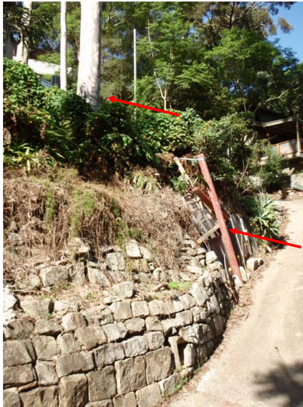
Photograph 1: Illustrating the location of the tree immediately above the failed section of retaining wall and adjacent embankment.
