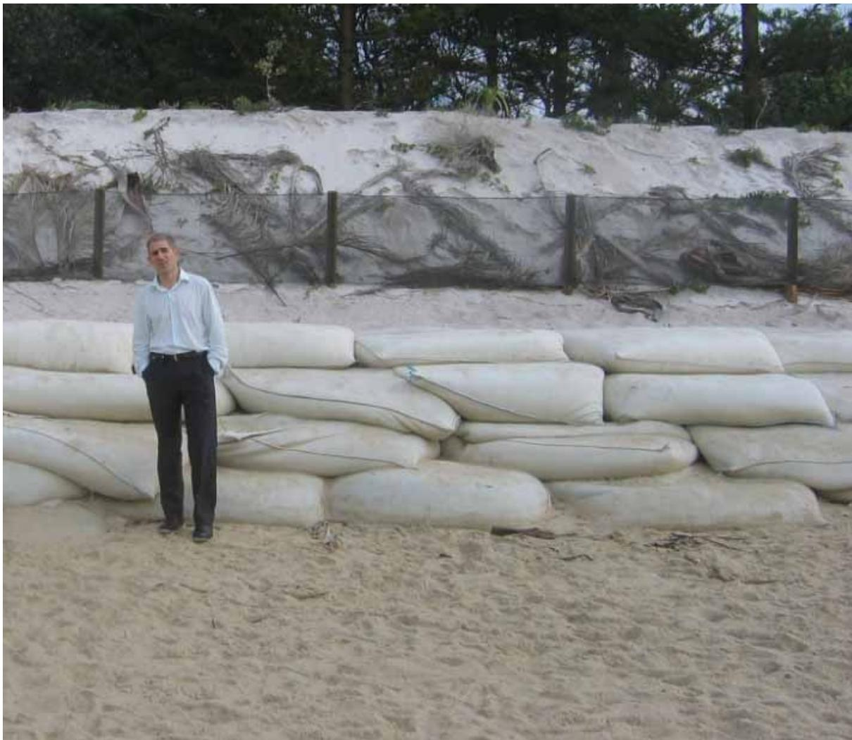
**Figure 2.2 – Geotextile sand container coastal protection works at Byron Bay**
