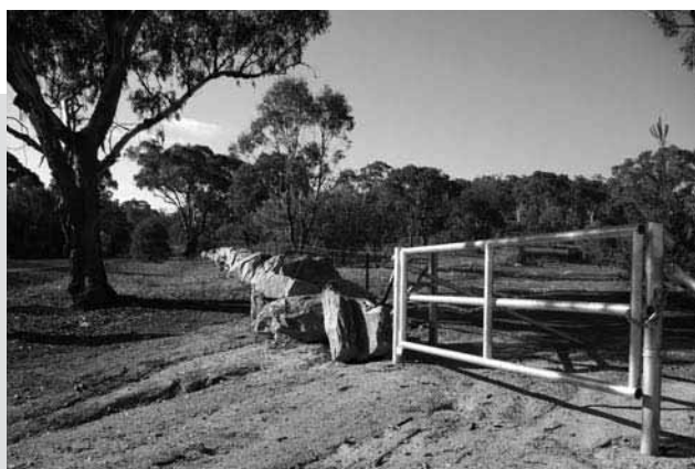
Sturdy gates and fences made from recycled materials were erected on the Mirrabee site in Queanbeyan.
