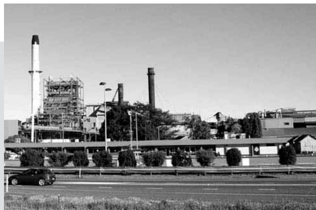
Condong Sugar Mill's new stack and boiler have replaced outdated equipment. The new plant will reuse treated effluent from the Murwillumbah sewage treatment plant, which will help improve water quality in Rous River.
