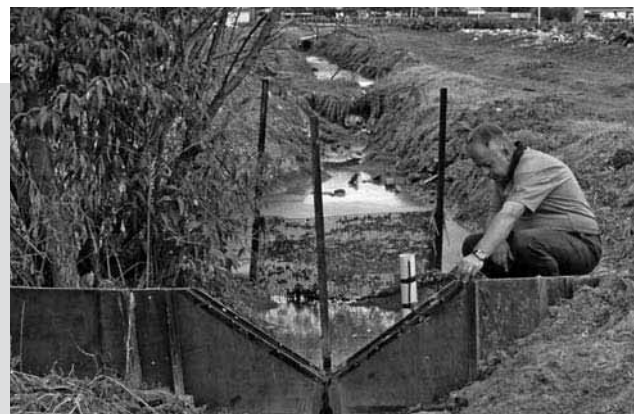
Richard Weber, DECC's project engineer, inspects the sampling weir that measures the amount of nutrient-rich runoff that the dam captures. The results show the dam and sophisticated pumping system DECC installed are successfully capturing runoff and preventing it from entering South Creek.
