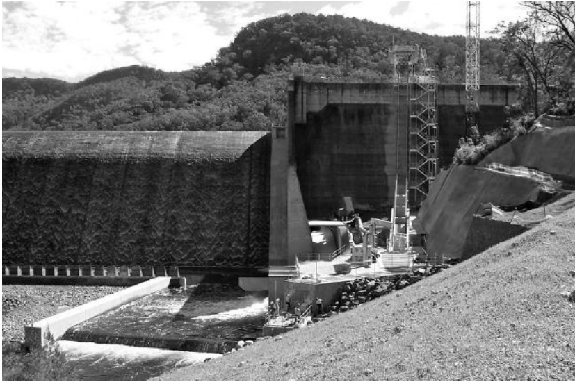
Tallowa Dam Fishway, showing fish passage provisions including the entrance, lift structure and hoist tower.
