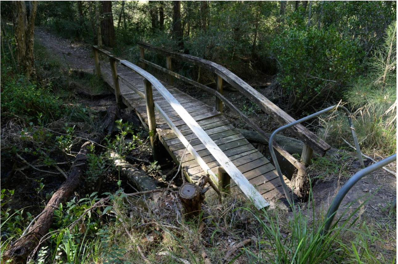
Photo 3: Vegetation around footbridge
