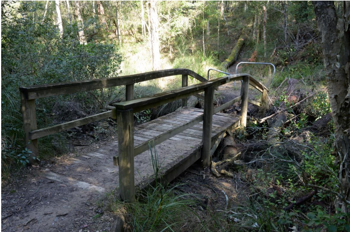
Photo 1: The Dawson River walking track pedestrian bridge
