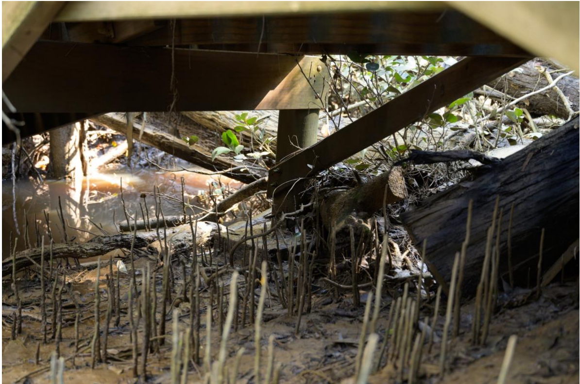
Photo 5: Underside of the pedestrian bridge at Dawson River walking track
