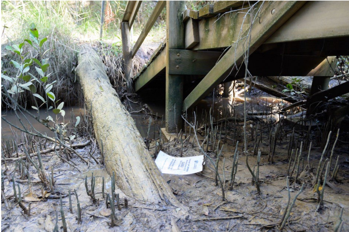
Photo 5 Grey mangrove pneumatophores within close proximity to the existing footings
