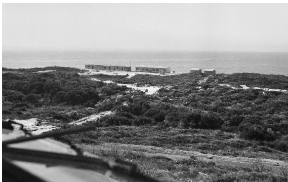
Buildings on flattened dunes to the east of the cemetery
