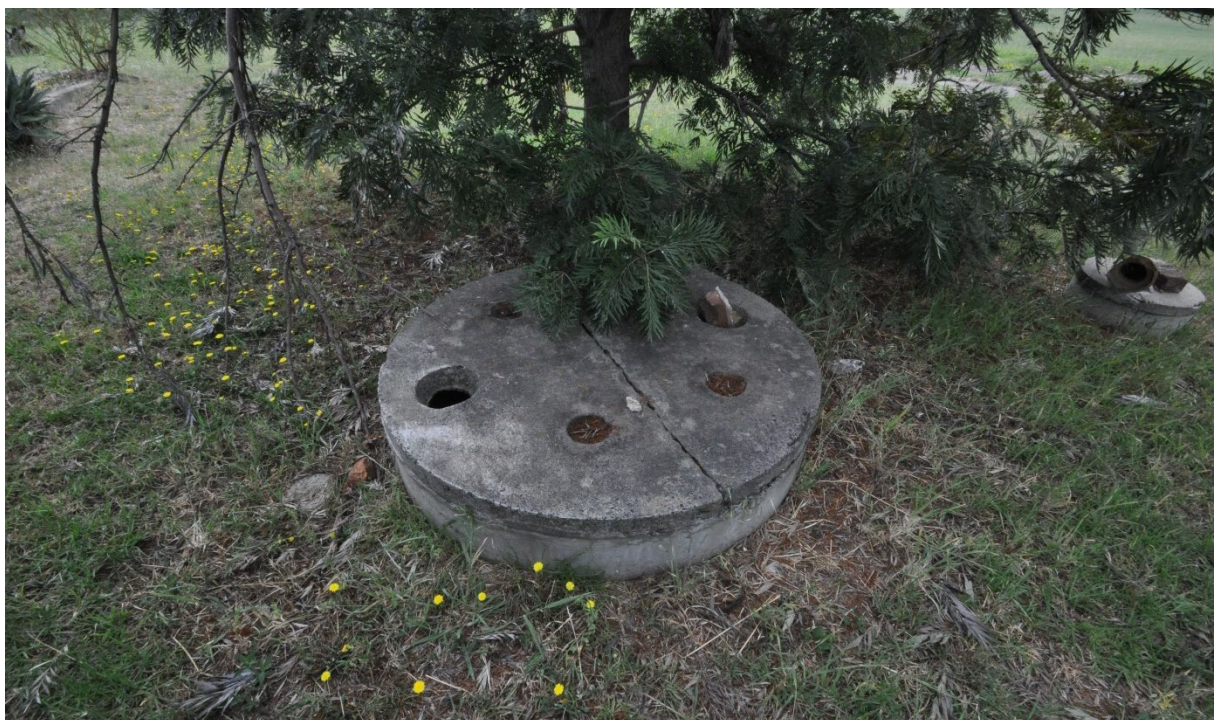
Figure 3.33 Concrete cover over a water cistern. This possibly replaced a former well. (Source: GML 2014)
