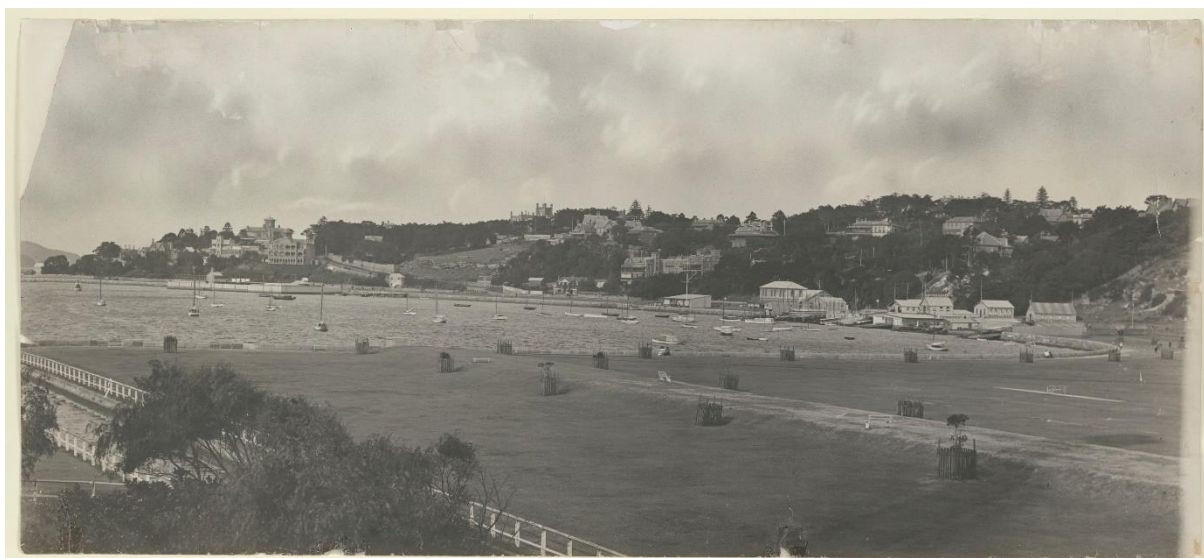
Figure 2.6 Panorama of Rushcutters Bay showing the park in the foreground and the boatshed and New Beach Reserve in the background, 1903–04. (Source: State Library of New South Wales, c11401_00_c(1).jpg)
