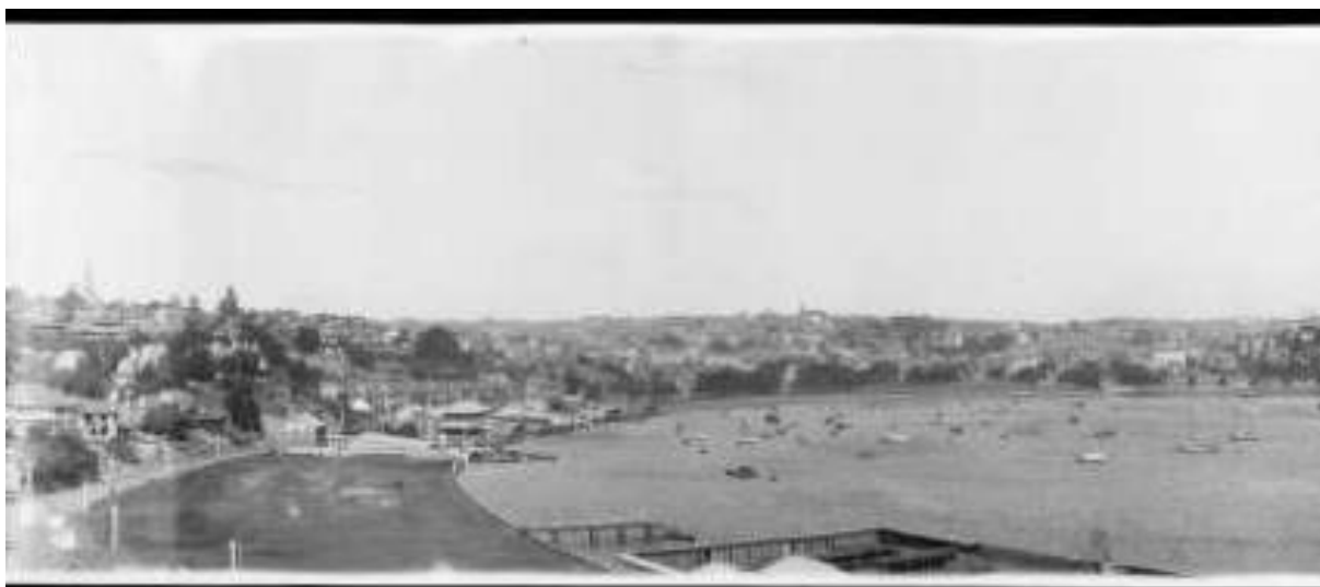
Figure 2.13 Part of 'Panorama of Darling Point and Rushcutters Bay, New South Wales', 2, c1917–1946, by EB Studios. The baths are visible in the foreground, right, next to New Beach Reserve (now Yarranabbe Park) edged by the seawall. (Source: National Library of Australia, ID number PIC P865/82/2 LOC Nitrate store)
