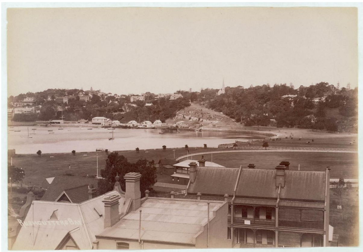
Figure 2.8 View east across Rushcutters Bay showing the oval and some plantings throughout the park, c1900–1910. Boatsheds and development are visible at a distance along the foreshore comprising the present-day Yarranabbe Park. (Source: State Library of New South Wales, a116074h)
