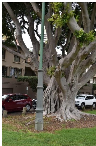
Figure 2.70 An early cast-iron sewer vent in the north of Yarranabbe Park, one of many found throughout the study area. (Source: GML, 2021)
