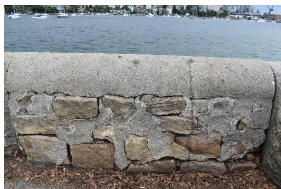
Figure 2.66 The stone repair to the seawall in the north of Yarranabbe Park. (Source: Ari Anderson, 2021)
