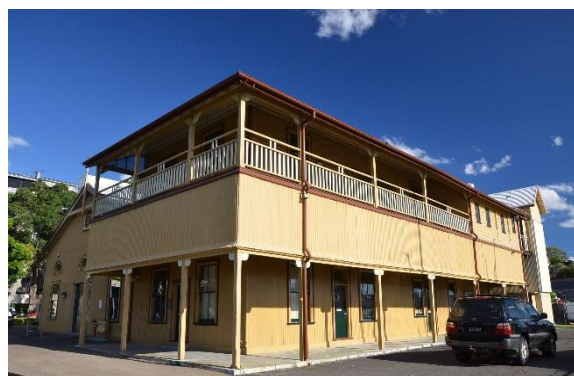
Figure 2.48 The former HMAS Rushcutter Drill Hall. (Source: Ari Anderson, 2021)
