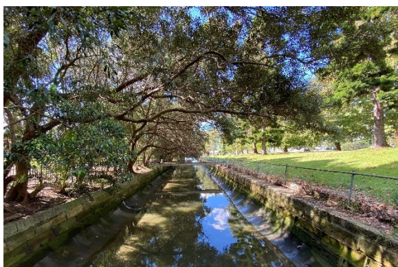
Figure 2.23 The stormwater channel in Rushcutters Bay Park.
