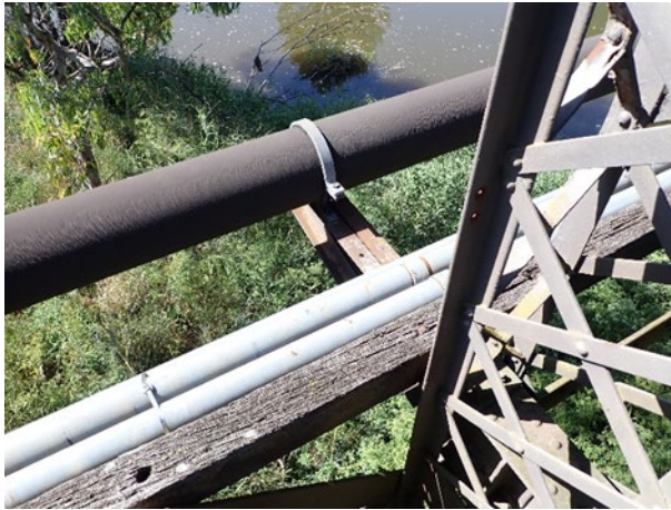
Figure 16 – Service pipes on upstream side view from bridge deck
