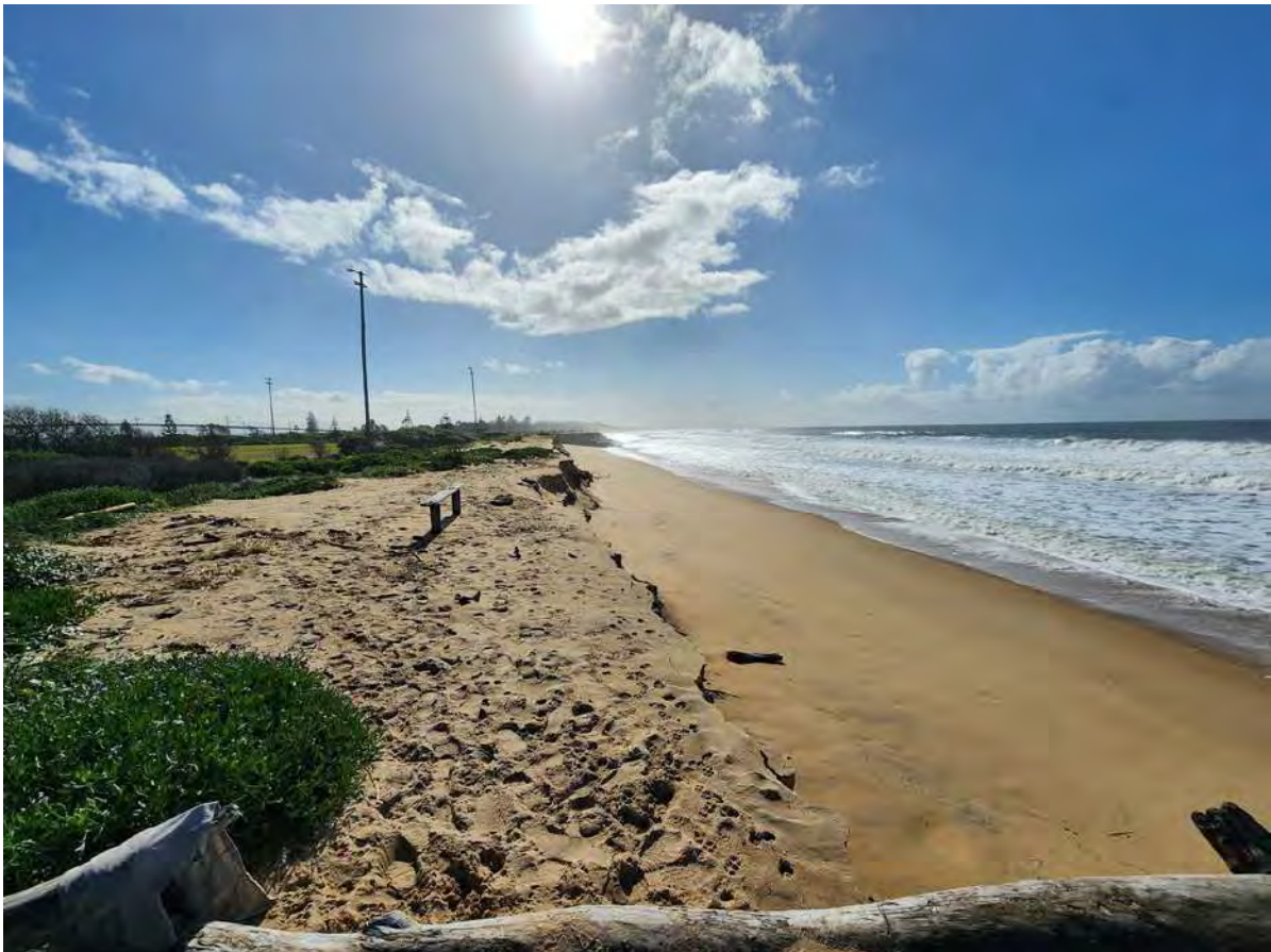
Coastal erosion at Stockton Beach, August 2024.
