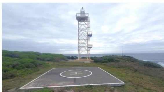
Photo 6-4: Steel lattice tower and helipad
