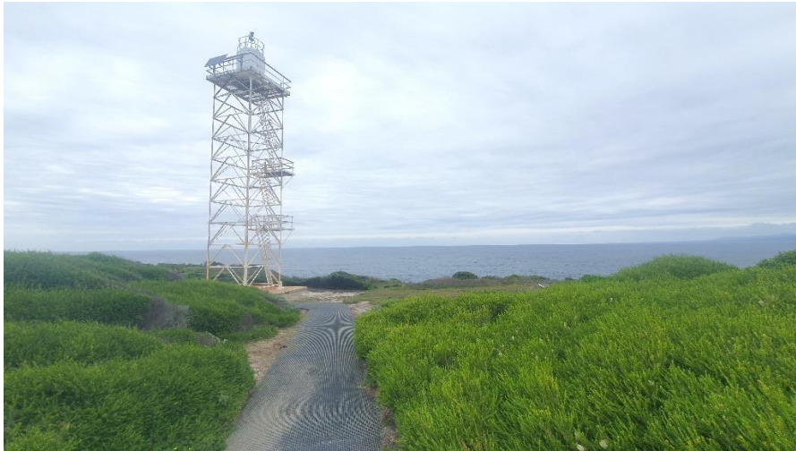
Photo 6-1: Steel lattice tower
