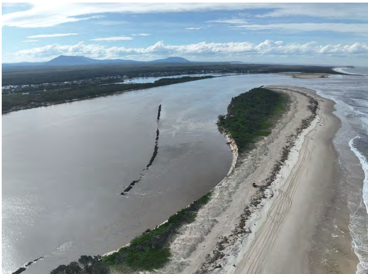
Figure 4: Damaged spur wall and breakthrough risk location.
