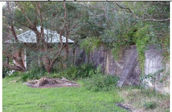
Photograph 11: Further evidence of the extensive levelling of the natural slope to accommodate the original armoury complex – only the buttressed retaining wall, a toilet block and the building foundations are still in evidence.
