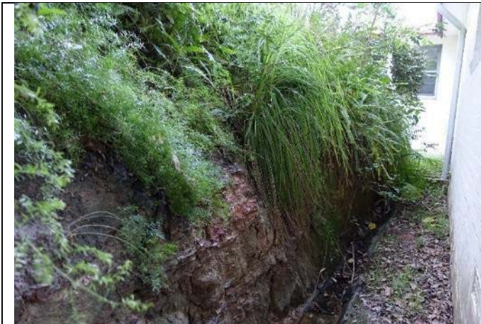
Photograph 8: Existing quarrying of the rock face at the rear of the building to rear a level surface for the building's foundations.
