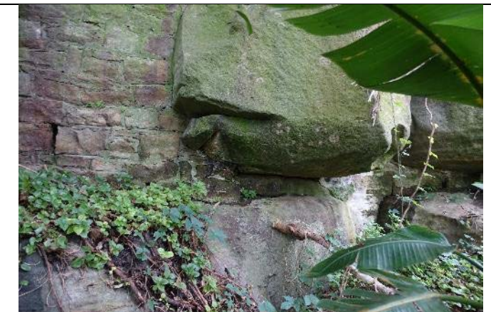
Photograph 21: Stone block wall set around sandstone bedrock on boundary with HMAS Watson
