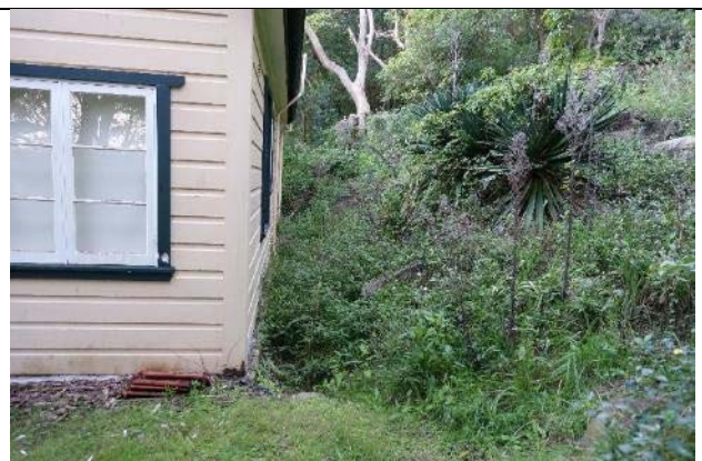
Photograph 7: Drainage channel at the rear of the building and the levelled surface at the foot of the natural slope.
