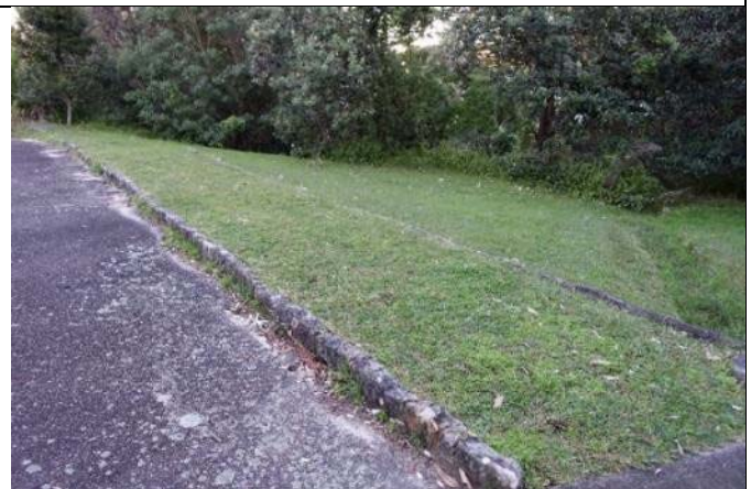
Photograph 4: Terracing channelling adjacent to the driveway on the north-western side of the Officers Mess circular drive
