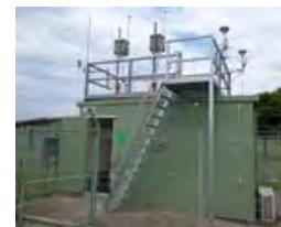
OEH Beresfield air quality monitoring station showing roof-mounted ASP samplers
