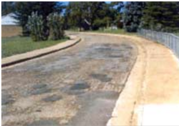
Repaired road at a salinity affected site
