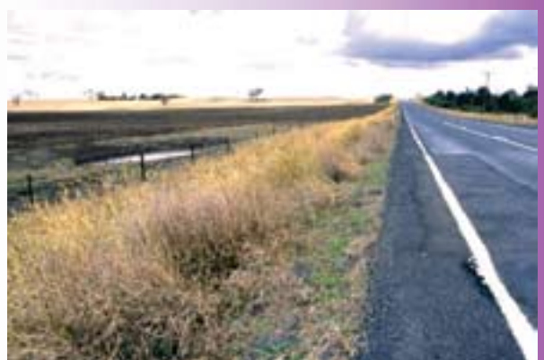
Repair of deformation in a rural road
