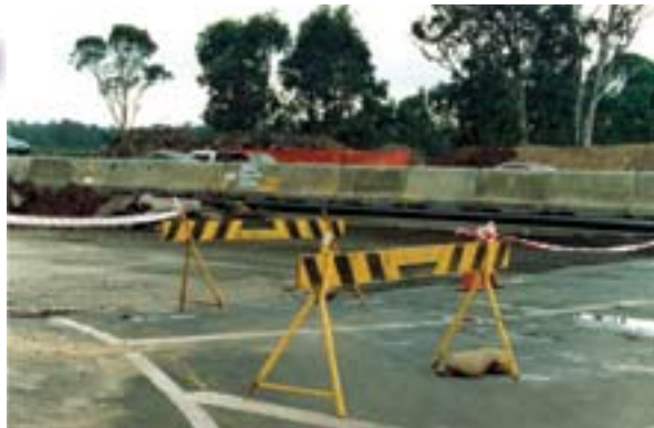
Road construction in layers
