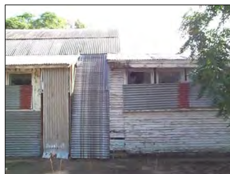
Figure 4.10: East hut junction with timber-framed kitchen. Also showing the SSAR hut cladding style. (Source – P Lofthouse)
