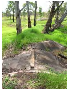
Figure 71 Remains of reinforced spillway.
