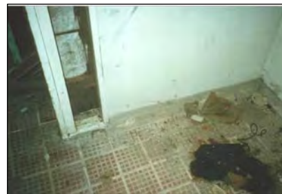
Figure 4.11: Kitchen flooring, with army partitions built over the original tiling. (Source – P Lofthouse)
