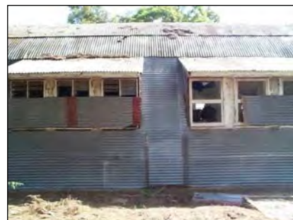
Figure 4.12: The two window styles, louvre and hopper (Source – P Lofthouse)
