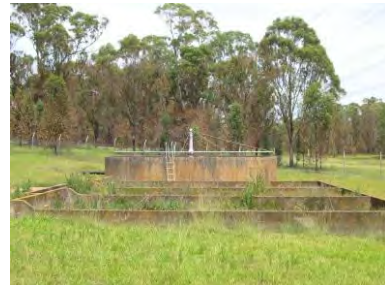
Figure 72 Settling Tanks
