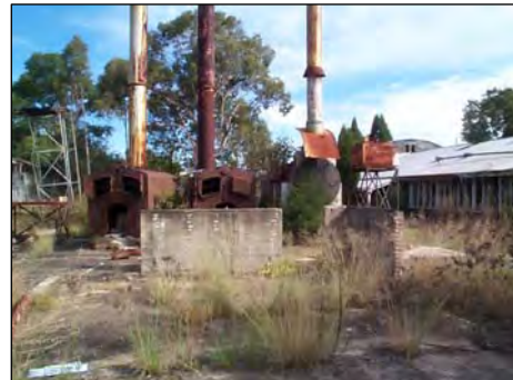
Figure 4.7: Boilers showing remnant walls from the boiler house, and tank stands (Source – P Lofthouse)
