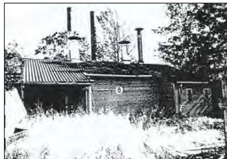
Figure 4.8: Boiler house in 1991 prior to demolition, showing vent cowlings. (Source – Edds, 1991)
