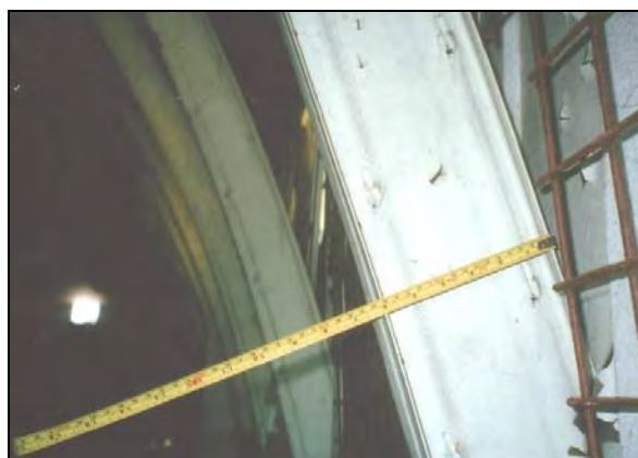
Figure 4.2: Structural “I” rib showing rivets and U section (Source - P Lofthouse)
