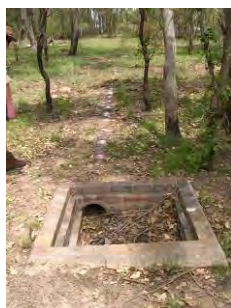
Figure 75 Brick inspection pit, vitreous clay pipes visible.
