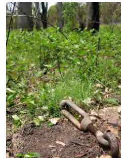
Figure 98 Turnbuckle and eyebolt fixed to a concrete pad provided tensioning to the cables. December 2005
