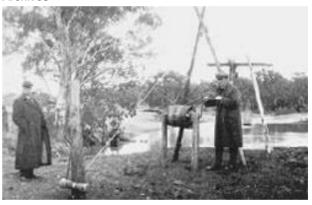
Figure 2.30 Lifting water, this winch and trestle was also used for wool bales and probably stores. Source: Yanga Archives
