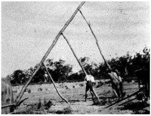
Figure 2.39 Erecting a pole, possibly for telegraph or power, Waugorah, 1925. Source: Museum of Victoria
