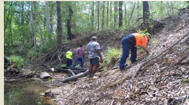
Erosion control on Busbys Creek
