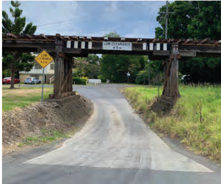
Photo 4: Road width - Frank Street viaduct
