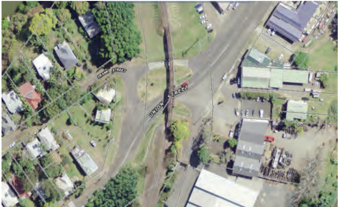
Figure 2: Aerial Photo Site 1 – Union Street, South Lismore
