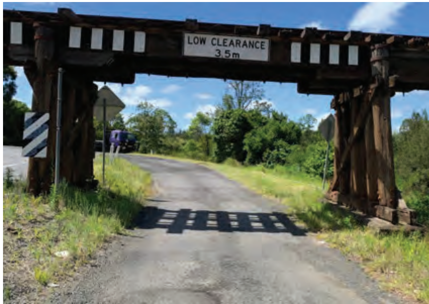
Photo 28: Road width – Alexandra Parade bypass viaduct
