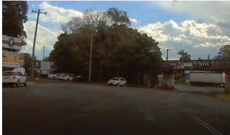
Photo 7: Industrial driveways north of Union Street viaduct
