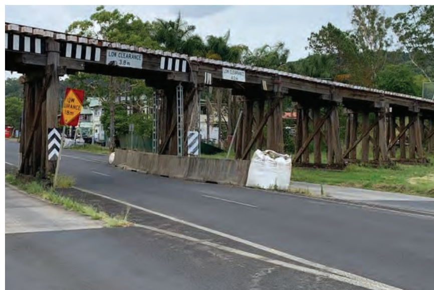
Photo 12: End of safety barrier (westbound) - Terania Street viaduct
