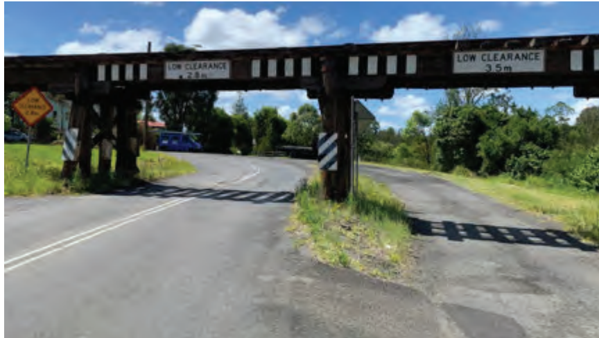
Photo 25: No edge lines and minimal edge clearance – Alexandra Parade viaduct
