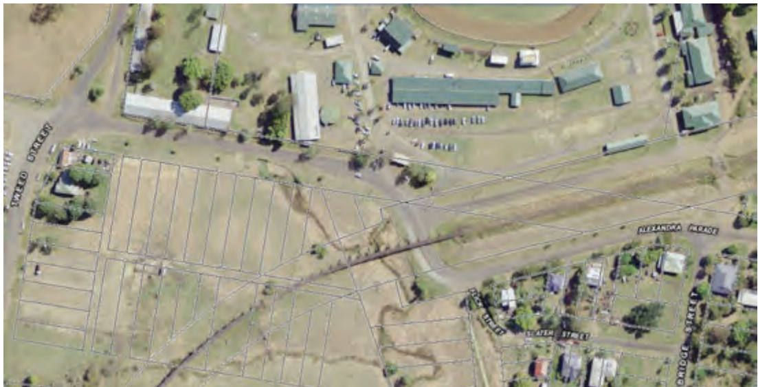
Figure 5: Aerial Photo Site 4 – Alexandra Parade, North Lismore
