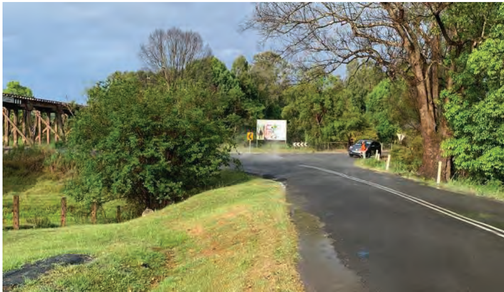
Photo 16: Inadequate definition of curve alignment – northbound approach to Winterton Parade viaduct
