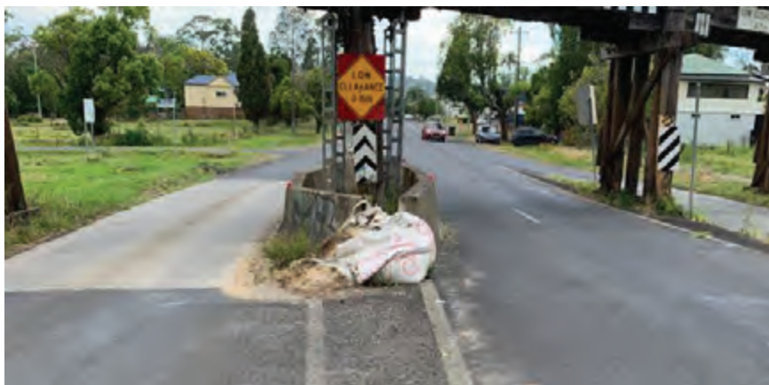
Photo 11: End of safety barrier (eastbound) - Terania Street viaduct
