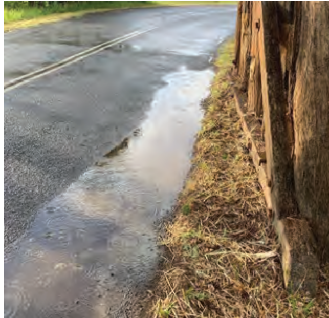
Photo 22: Roadside drainage at Winterton Parade viaduct
