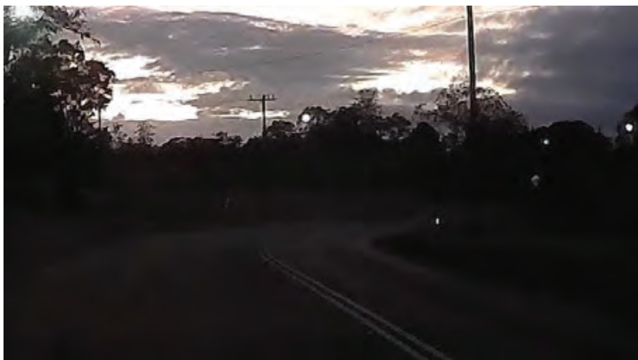
Photo 33: Night visibility - eastbound approach to Alexandra Parade viaduct
