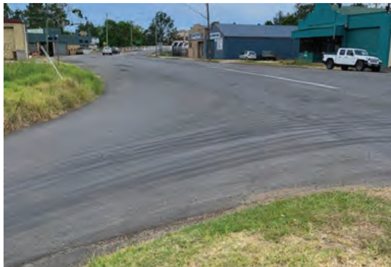
Photo 5: Lack of intersection controls - Frank St/Union St intersection
