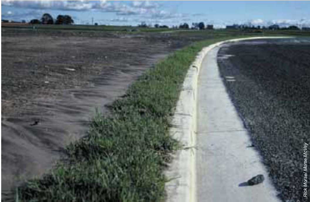
Turf strips control sediment in low flows
