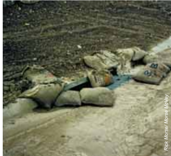
Sandbags can control sediment effectively [left] or be a hazard if neglected [right]
