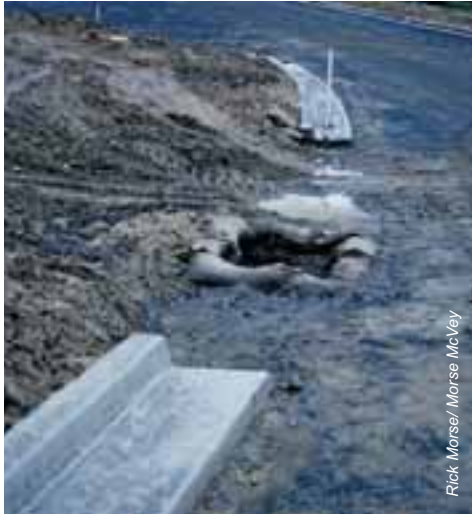
Sandbags can control sediment effectively [left] or be a hazard if neglected [right]
