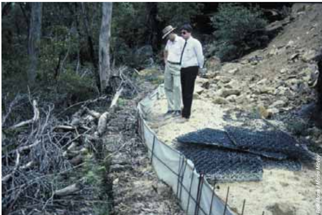
Building materials stockpiled with sediment fence
