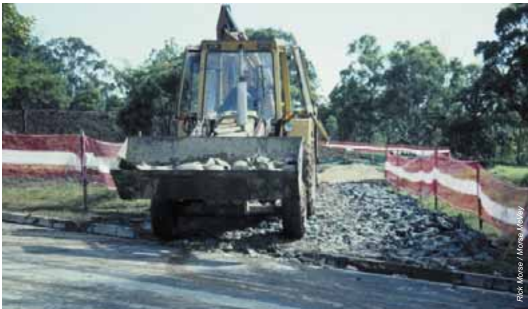
Controlled access to a site reduces erosion and controls sediment
