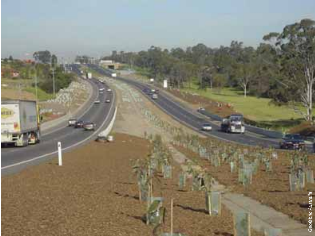
Jute matting stabilises newly planted area
