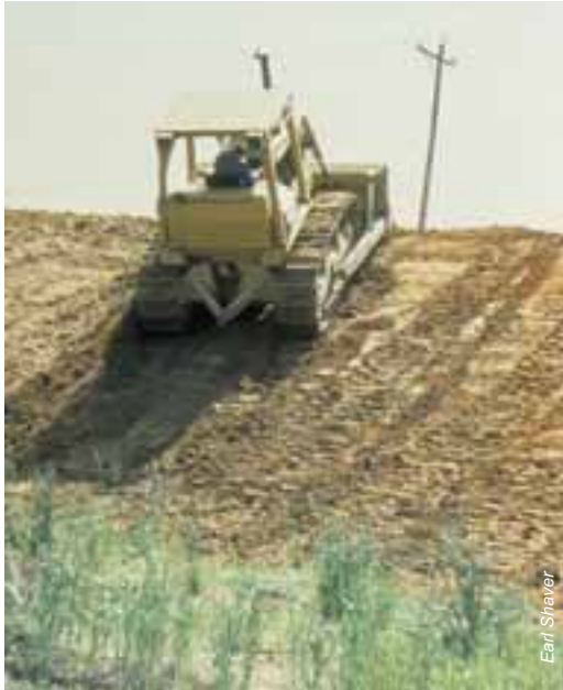
Track walking using a dozer [left] helps reduce erosion and encourage vegetation to establish [right]
