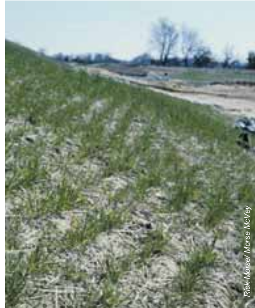
Track walking using a dozer [left] helps reduce erosion and encourage vegetation to establish [right]
