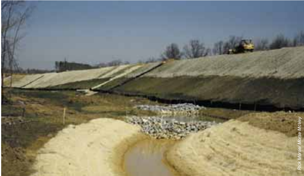
Progressive revegetation and stabilisation of batter
