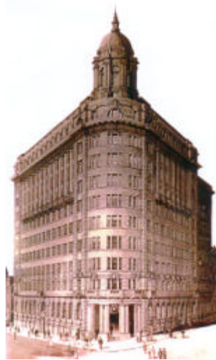
Figure 4: An Archival print of the Wales Building, looking North at the junction of Pitt, Hunter, and O'Connell Streets.
