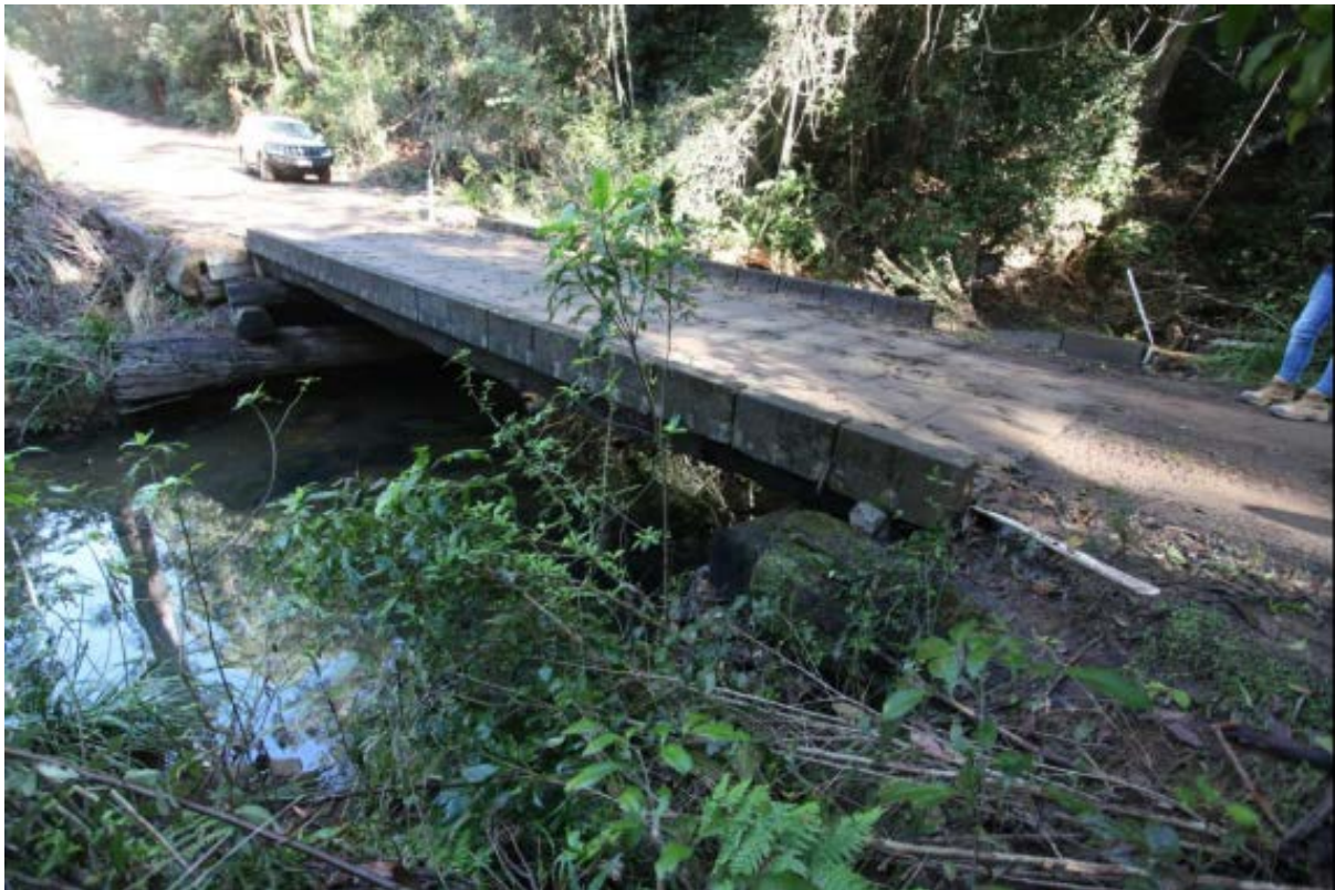
Figure 6 Buds Crossing Road Bridge (Everick 2021b)
