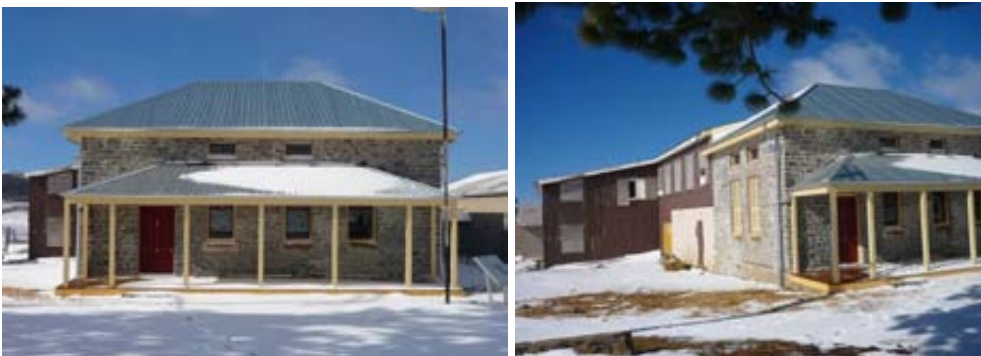
Front of Kiandra Courthouse following completion of works Photos: DECCW
