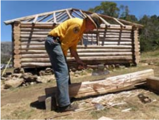
Peter Scobie dressing a slab, Pretty Plain Hut rebuilds. Photo: Megan Bowden DECCW
