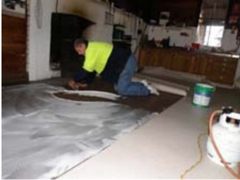
Installing new flooring Pines Cottage Currango Homestead. Photo: Megan Bowden DECCW
