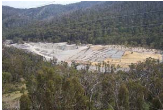
Rehabilitation works at Snowy Adit. Photo DECCW
