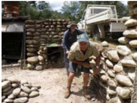
Gary McDougal & volunteer reconstructing Dr Forbes hut. Photo: Megan Bowden DECCW
