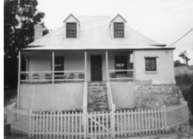
Ivy Cottage, Hartley Village, an example of the many state significant items uncovered by the State Heritage Register Project.
