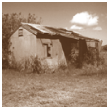
Mission Building, Ulgundahi Island. Photograph by Adell Hyslop.
