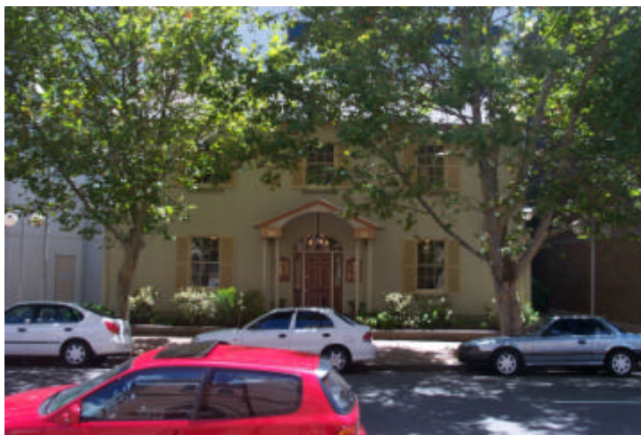
Figure 6: Macquarie Street façade of 'Kia Ora' at present.
