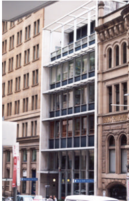
Figure 13: Liner House – now Moran House.
