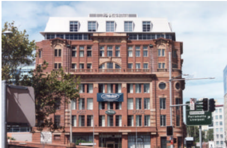
Figure 9: Northern façade of the former Parcels Post Office, now Medina Apartments.
