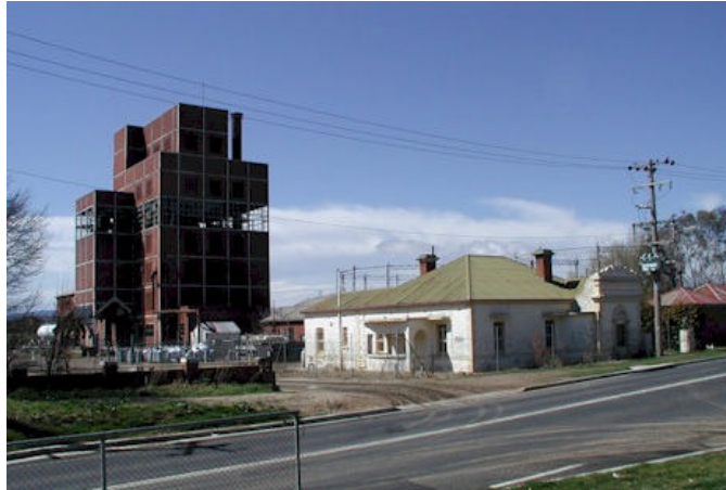
Gasworks, Bathurst, NSW, 1887. The first municipally-owned works in Australia.
