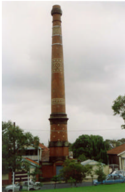
Sewer Vent, Lewisham
