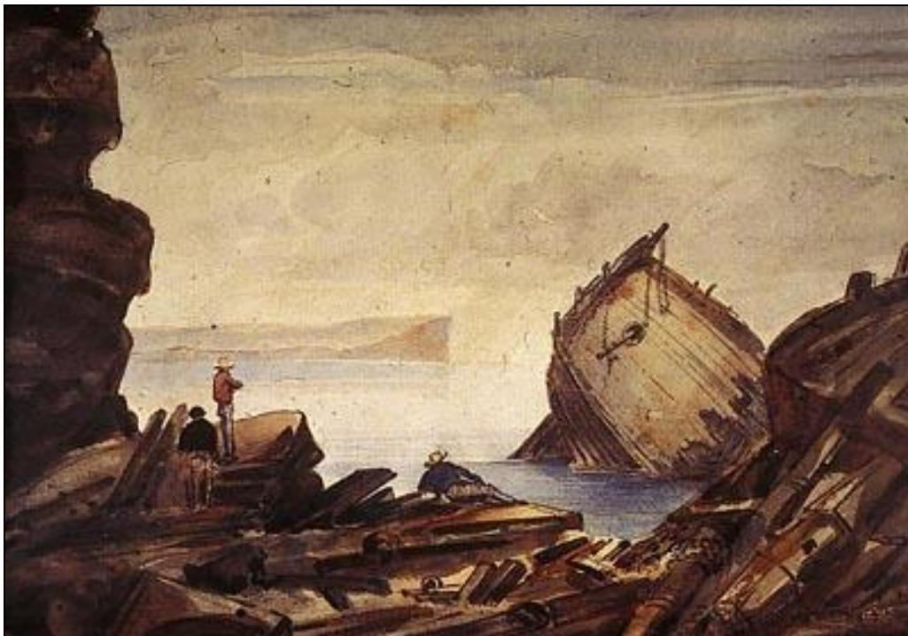
Figure 3 - "Wreck of the Edward Lomb [sic]", water colour attributed to Conrad Martens. Undated. Dixon Gregory Collection, Mitchell Library. Sydney.
