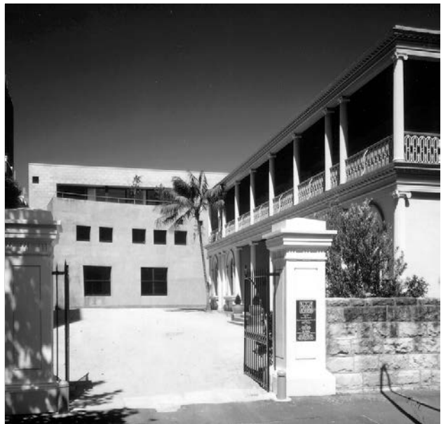
'Tusculum', Potts Point. A modern extension of a heritage building can be successful if carefully designed in terms of proportions and form. The Royal Australian Institute of Architects (NSW) added this modern office building to the rear of its heritage property. Photo: Patrick Bingham-Hall.
