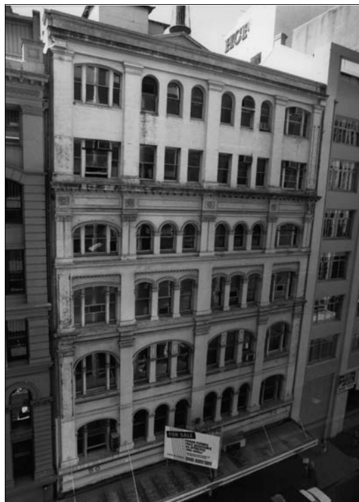
York House, Sydney is among significant city buildings that are being adapted for re-use to capitalise on their heritage value whilst providing modern accommodation and facilities. It forms part of an historic streetscape of 19th century commercial buildings terminated by a view of Sydney Town Hall. Proposals are being considered that retain its interior construction and rear address to an historic laneway while allowing some additional floors. Photo: Stuart Humphreys.
